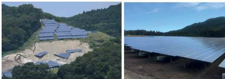
A solar power plant in Hyogo Prefecture. This plant partially collapsed during the Western Japan Heavy Rain Disaster of 2018. ©Nikkei BP.
