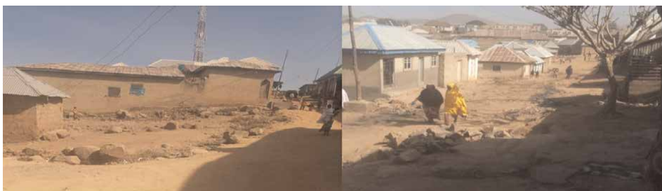
Figure 9. Nocturnal developments without basic infrastructure i.e without sewage disposal, drainages & Children Play ground.
