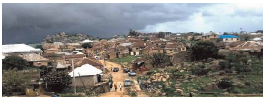
Figure 3. Kabong Settlement with Haphazard Developments within a difficult Topography.
