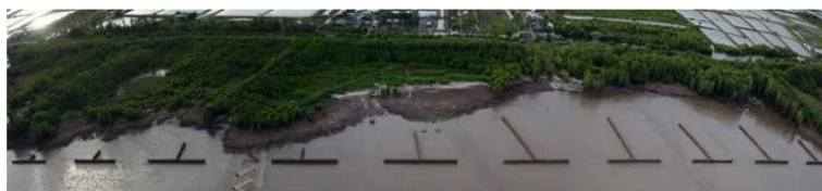
Figure 3. Placement of T-fences to minimise lee erosion (Bac Lieu Province, Viet Nam, photo Cong Ly and G.E. Wind 2013).
