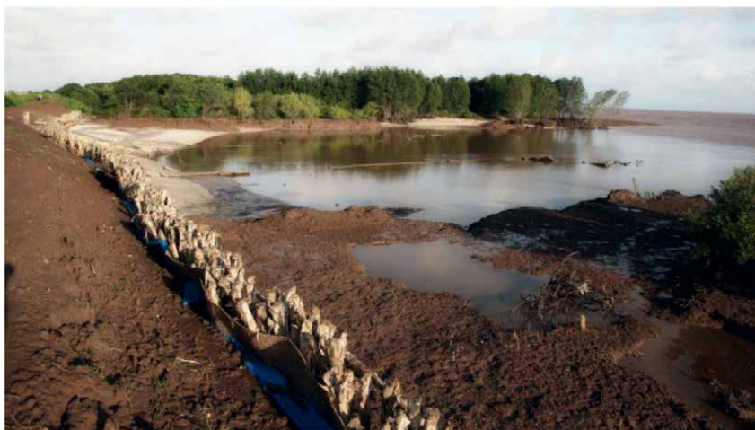
Figure 1. Eroded tidal flat. The dyke protection with concrete and Melaleuca fences failed to stop the erosion (Nopol, Soc Trang Province, Mekong Delta, Viet Nam, photo K. Schmitt 2010).
