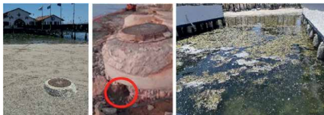
Figure 3. Sewage leaks make a significant contribution to nutrients, in addition to numerous more dangerous pollutants. This can be seen in this figure and is directly related to the algae growth on the shore of the beaches. (Mar Menor, Murcia, Spain).
