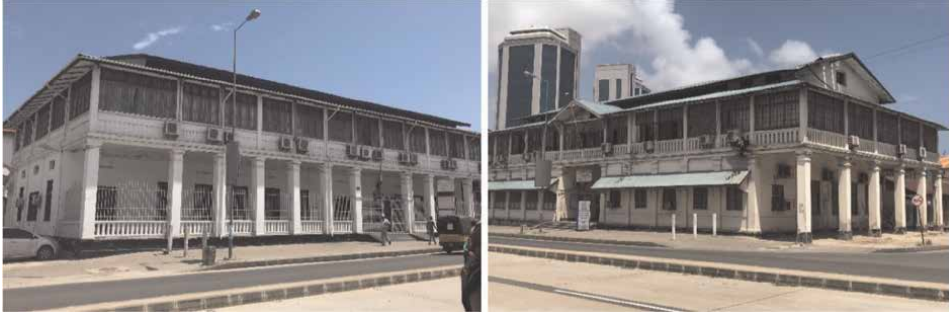
Figure 1. Series of German buildings with balconies covered to increase the floor plan area.
