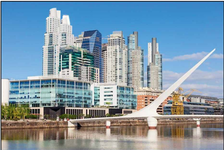
Figure 6. Puerto Madero, Buenos Aires.
