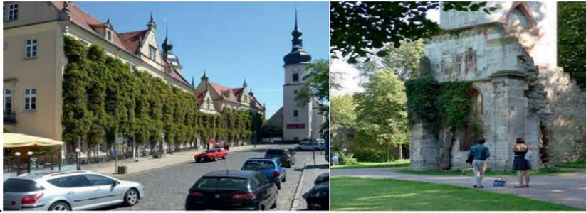
Figure 10. Full-surface facade greening with wisteria on climbing supports, town hall Riesa / Saxony, ancient ivy in the nature park on the Ilm river in the Templar hall, Weimar/Thürigen [36]. https://www.fassadengruen.de/en/classicism-and-building-greening.html
