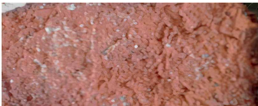
Figure 10. Brick after efflorescence test.
