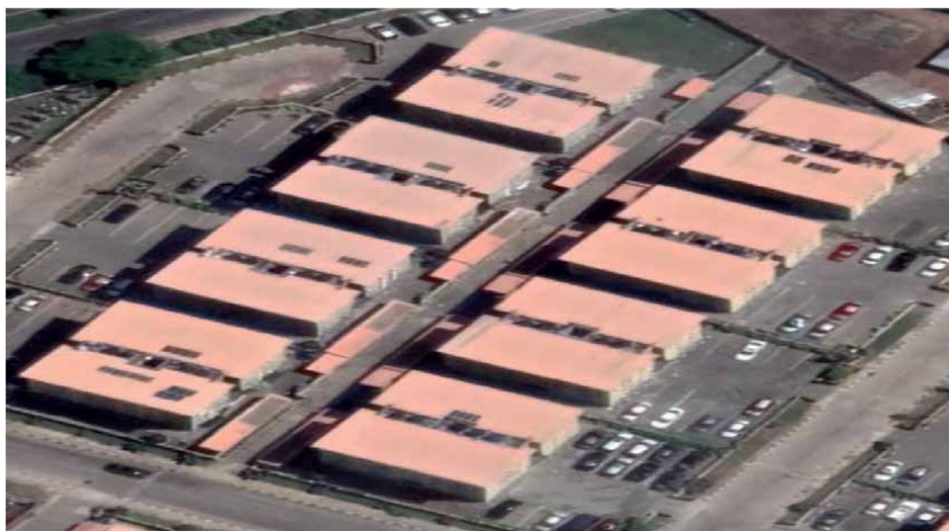
Figure 3. A Section of the Lagos HOMS layout showing the closeness of the blocks. Source: [92].
