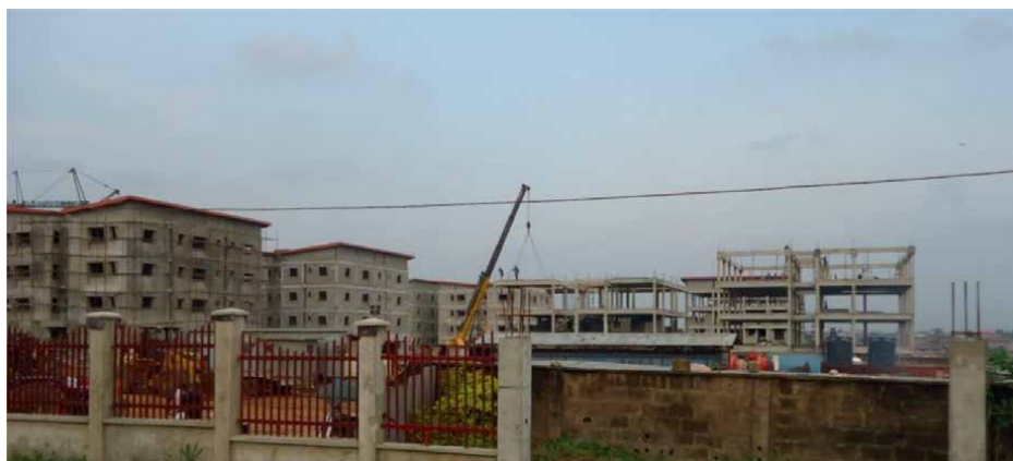
Figure 4. Hoisting of Prefabricated Slabs. Source: [91].
