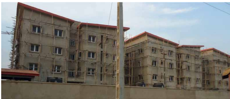
Figure 2. Compact arrangement of the blocks under construction. Source: [91].
