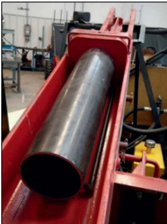
Figure 19. Horn 2" tube well installation drive sleeve positioned in hydraulic ram channel [10].
