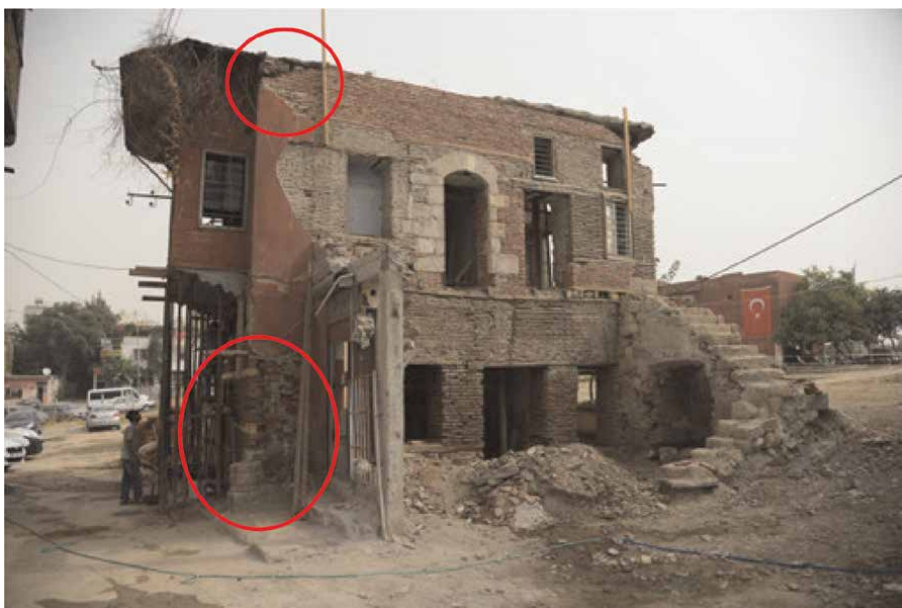
Figure 9. Traditional Tepebağ house with inventory number 63, west view.
