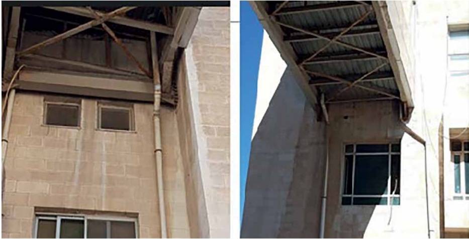
Figure 2. The connecting steel sky bridge from below.
