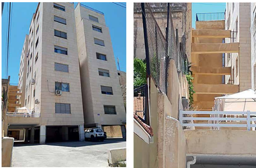
Figure 10. A building connected to a nearby wall by several beams at different floor levels, Amman, Jordan.
