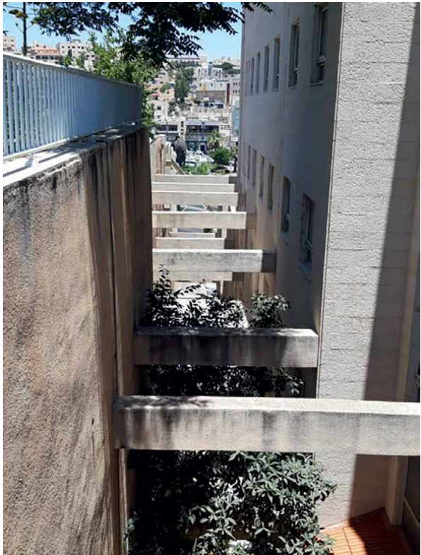
Figure 9. A multi-story building connected to the nearby wall by beams at several floor levels, Amman, Jordan.
