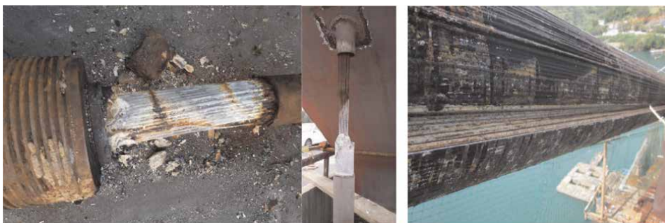
Figure 1. Corrosion and fatigue damage of cable-stayed bridges in mountainous areas with cable-stayed cable, suspension cable, and main cable.
