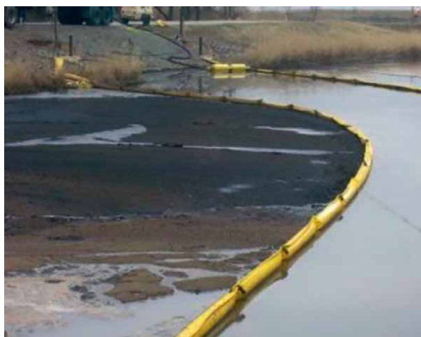
Figure 3. Use of the oil containment boom [28].
