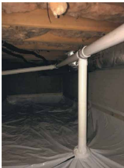
Figure 6. Example of sub-membrane suction system [23].
