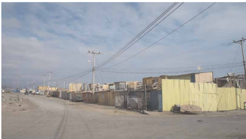
Figure 19. Self-construction and informal settlements that defy construction and safety standards.
