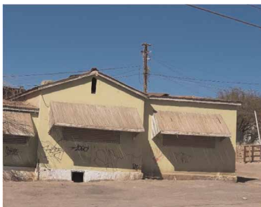
Figure 22. Façade with fixed shade house vernacular house of María Elena.
