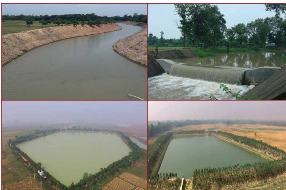
Figure 3. Surface water augmentation by (a) re-excavated canal, (b) cross dam (check dam) in the re-excavated canal, (c) re-excavated pond and (d) re-excavated natural beel utensils (source: [22]).
