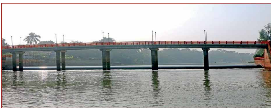
Figure 6. A rubber dam was constructed across the river (source: [12]).
