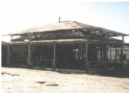
Figure 20. Case of a house in the Chacabuco saltpeter office, with a shaded corridor around the perimeter and a double ventilated roof and shading system.
