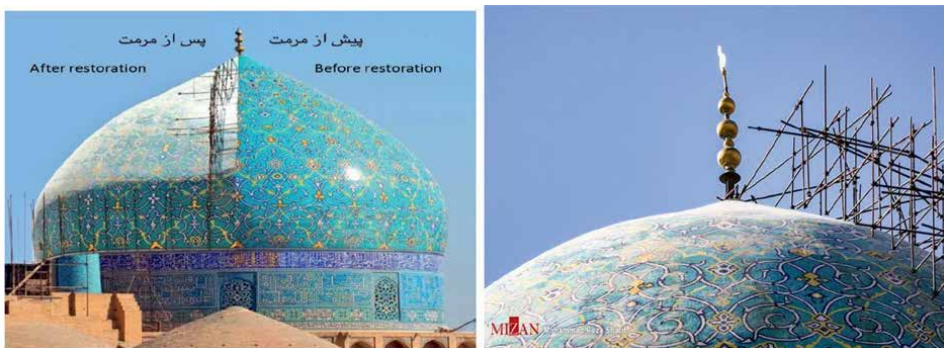
Figure 3. Before and after the restoration of the Shah dome of Isfahan. Source: [3, 13].
