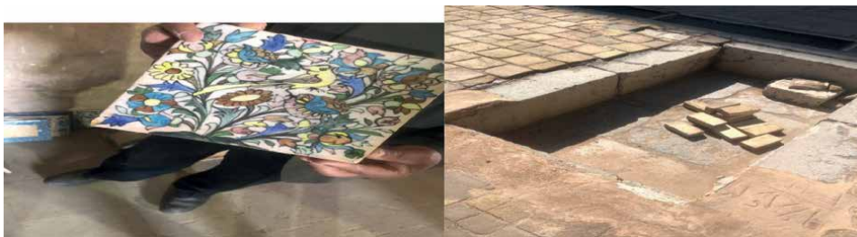
Figure 7. Repair and maintenance status of NAGHSHE-JAHAN Square. Source: [7, 27].
