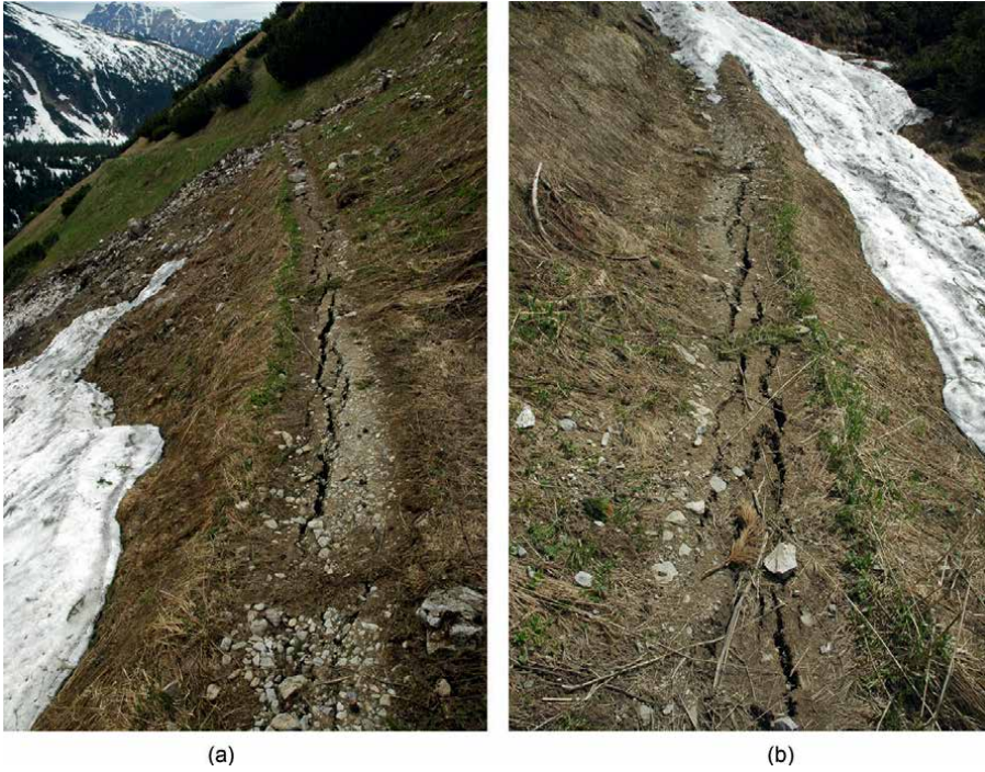
Figure 23. Expansion cracks on the hiking trail after melting of the snow field on the SW slope of the Belianské Tatras (Hreško, 2009).
