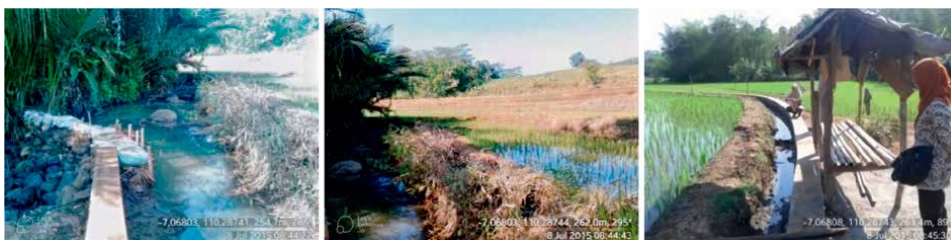
Figure 9. The secondary irrigation channel has a disconnected position with a tertiary channel in Trisobo Village, Boja District.
