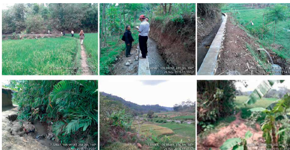
Figure 11. The location of the irrigation network is in Bendosari Village, Plantungan District.
