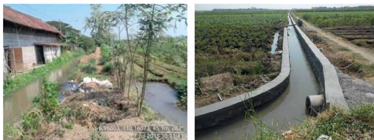
Figure 4. Secondary irrigation channels in Gubugsari Village, Pegandon District (not yet repaired), and tertiary irrigation networks in Gubugsari Village, Pegandon District.
