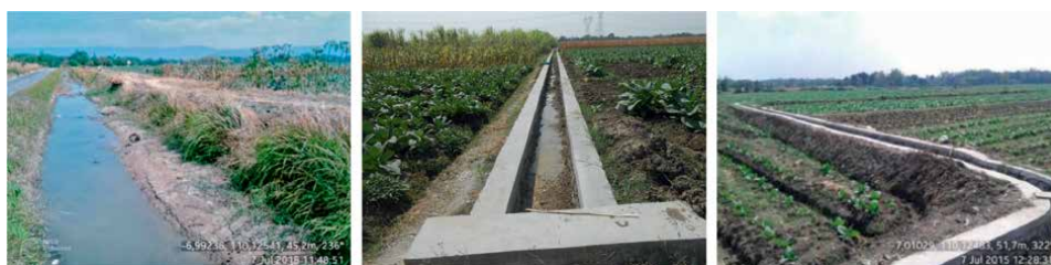
Figure 5. Secondary (no restoration) and tertiary channels in Galih Village, Triharjo Village, Gemuh District.
