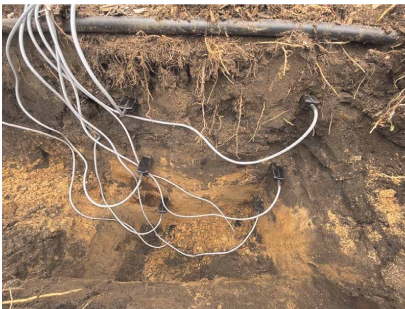
Figure 3. Installed FDR soil moisture sensors in a blueberry field (west olive, MI, USA).
