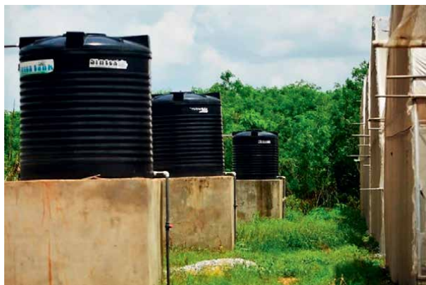
Figure 9. Water tanks are elevated above the level of the field to allow for the natural flow of water and nutrients.
