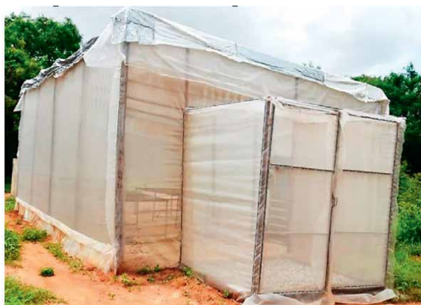
Figure 2. Greenhouse of Institute of Applied Science and Technology (IAST), University of Ghana built from bamboo.
