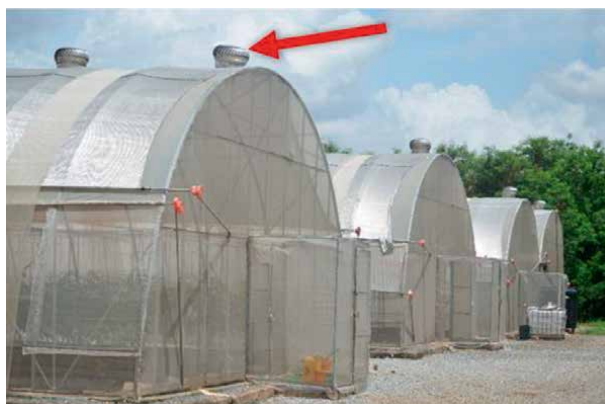
Figure 4. Circulation fans (chimney) are fixed on greenhouses of IAST to regulate the climatic conditions in the greenhouse.
