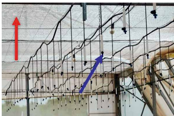
Figure 5. Misting/fogging and hosing (blue arrow) are used to regulate the climatic conditions as well a shade net (red arrow) is used to reduce the intensity of solar radiations in the greenhouse.
