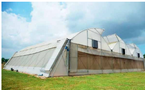
Figure 1. Greenhouse of West Africa Center for Crop Improvement (WACCI), University of Ghana built from galvanized metals including steel or aluminum.
