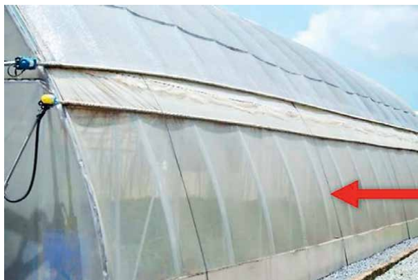
Figure 3. Fixing of side nets (indicated with the arrow) to provide natural ventilation.
