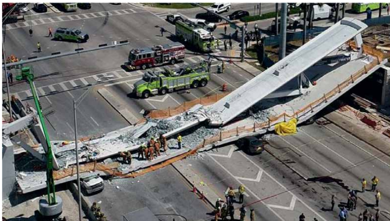
Figure 8. Collapsed pedestrian bridge Miami, FL. CC BY-SA 3.0.
