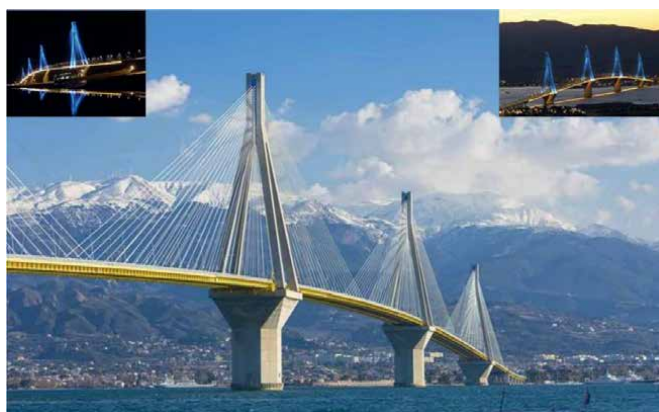
Figure 4. Cable-stayed bridge Rio Antirrio Bridge in Greece. Opened 2004 length 2.8 km. CC BY-SA 3.0.
