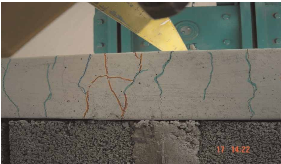
Figure 2. Evolution of cracking as the load was applied.
