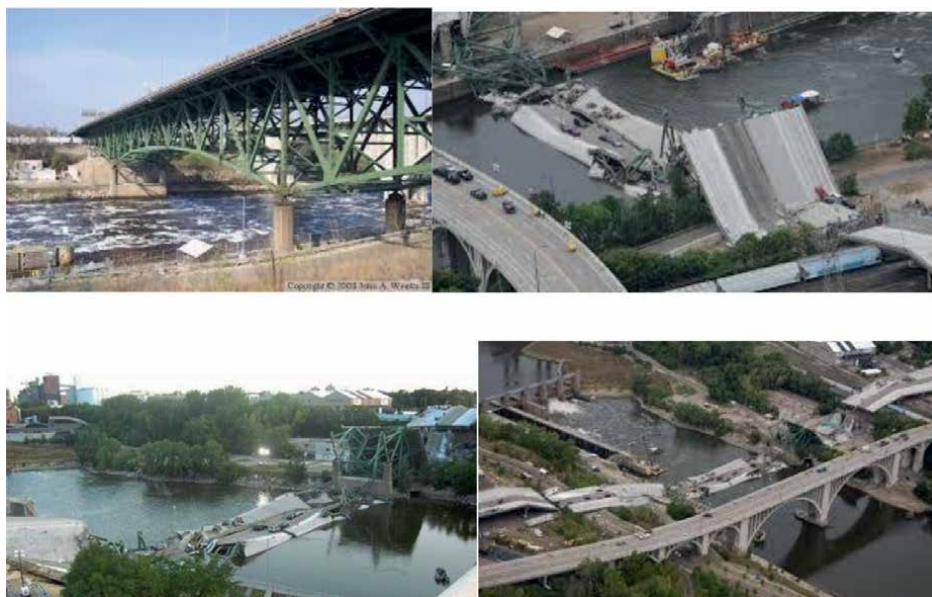
Figure 9. I-35 W Mississippi River Bridge collapse. CC BY-SA 3.0.
