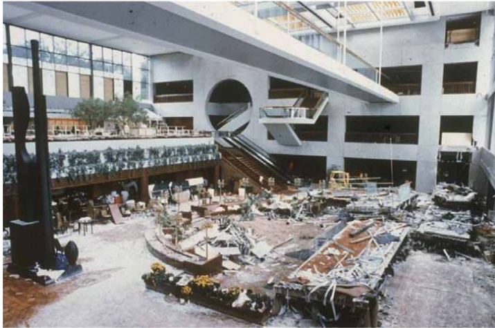
Figure 10. Fourth and second floor skywalks falling to the atrium. CC BY-SA 3.0.
