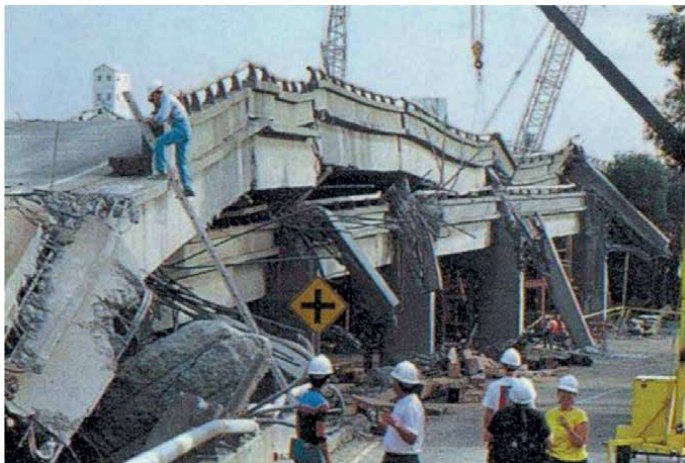
Figure 12. Collapse of the I-880 freeway in the 1989 Loma Prieta earthquake. CC BY-SA 3.0.
