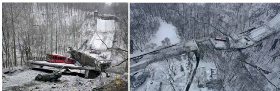
Figure 7. Collapsed Pittsburgh bridge January 2022. CC BY-SA 3.0.
