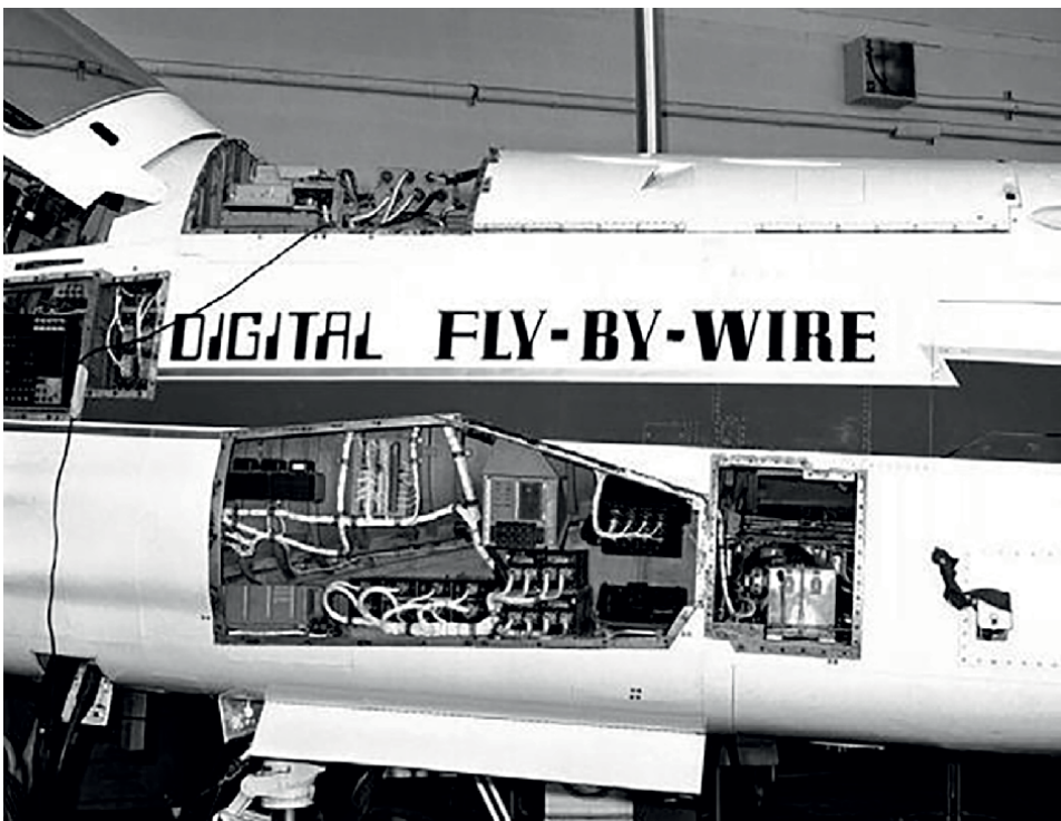
Figure 6. Digital fly-by-wire system [14].
