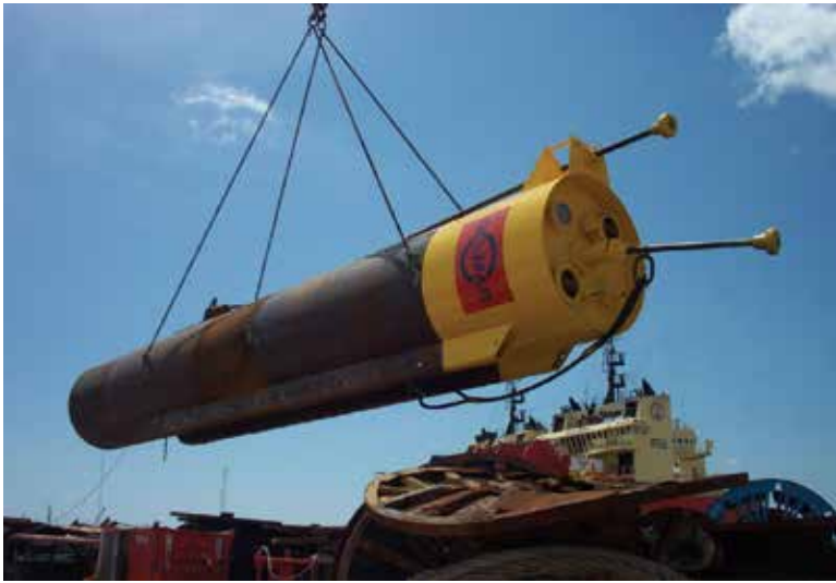
Fig. 10. Suction Anchors for an offshore platform being transported to site in the Gulf of Mexico (Courtesy Prof Aubeny, TAMU).
