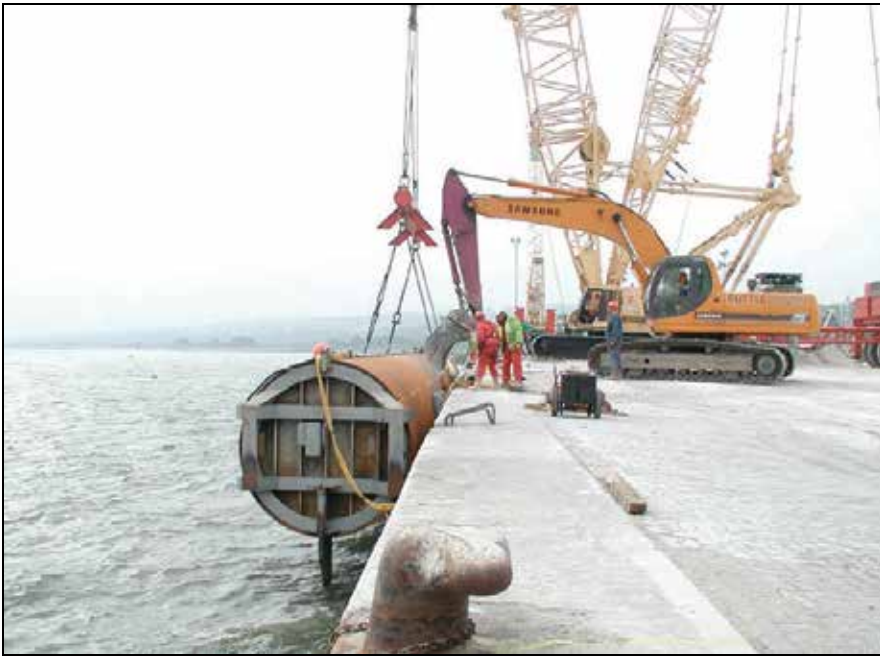
(a) Monopile being floated out to site.
