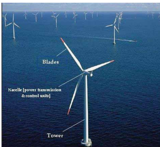
Fig. 1. Offshore horizontal-axis wind turbine
