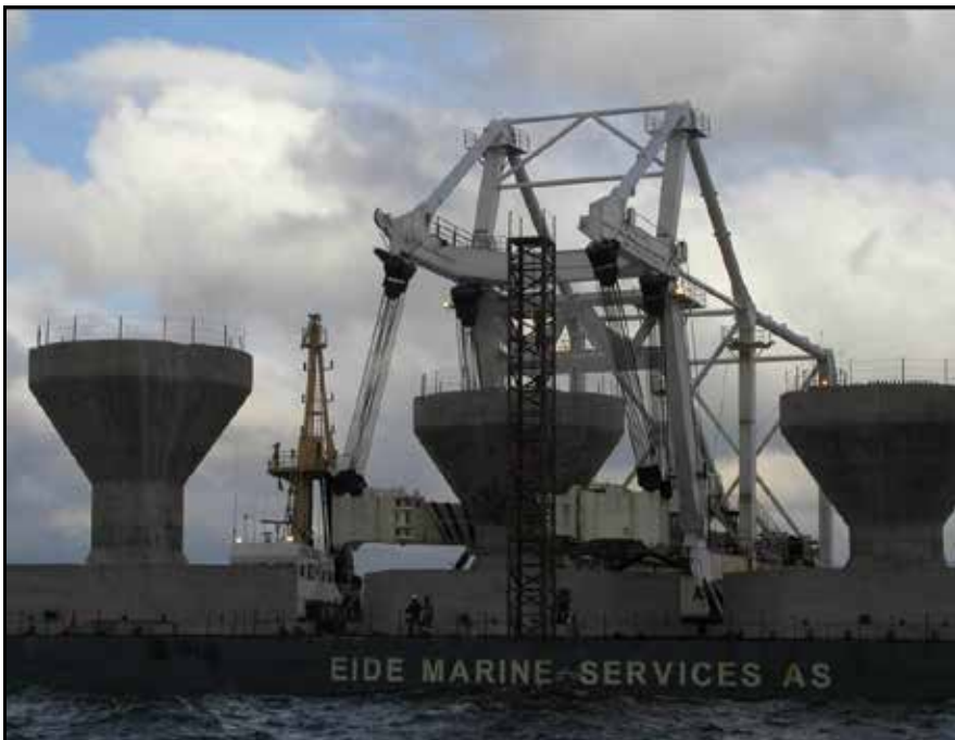
(b) Gravity Bases being lowered from barge
