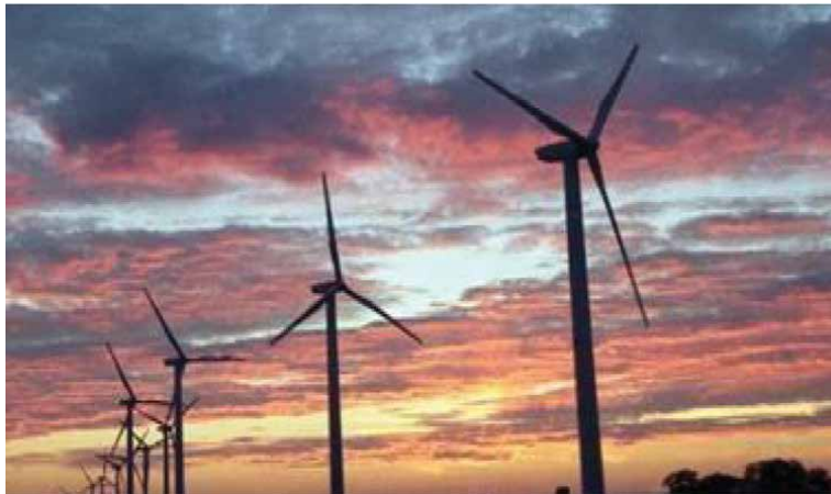
Figure 7. Wind energy generating system [14].
