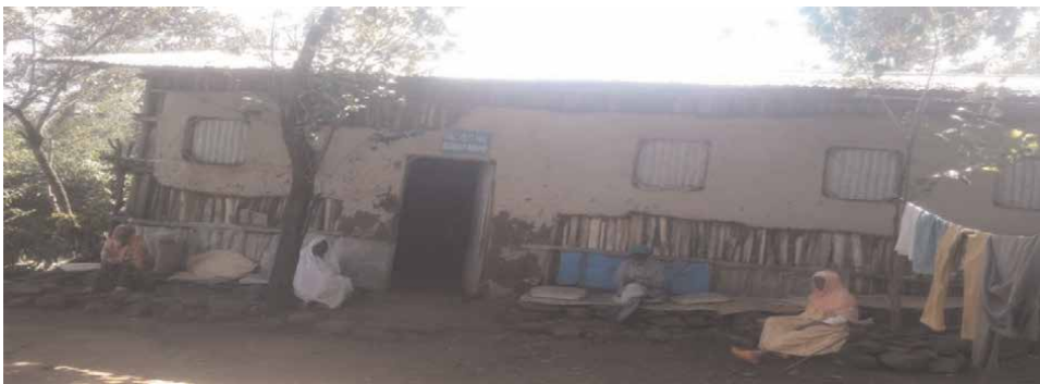
Figure 6. The community elder care house external picture (photo of the author).
