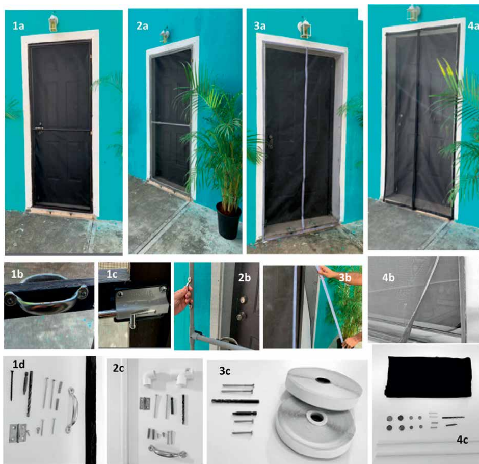
Figure 1. Different options and materials for the installation of house screening other than aluminum: (1a–1d) wood, (2a–2c) polyvinyl chloride plastic (PVC), (3a–3c) velcro and (4a–4c) magnets.
