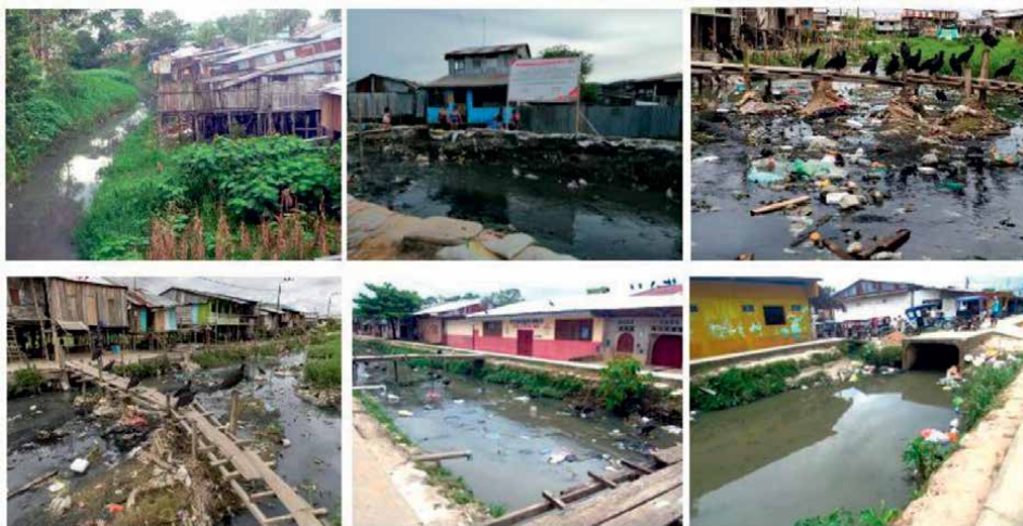
Figure 2. Typical open-air sewage systems in Iquitos city and other main cities of the Peruvian Amazon.
