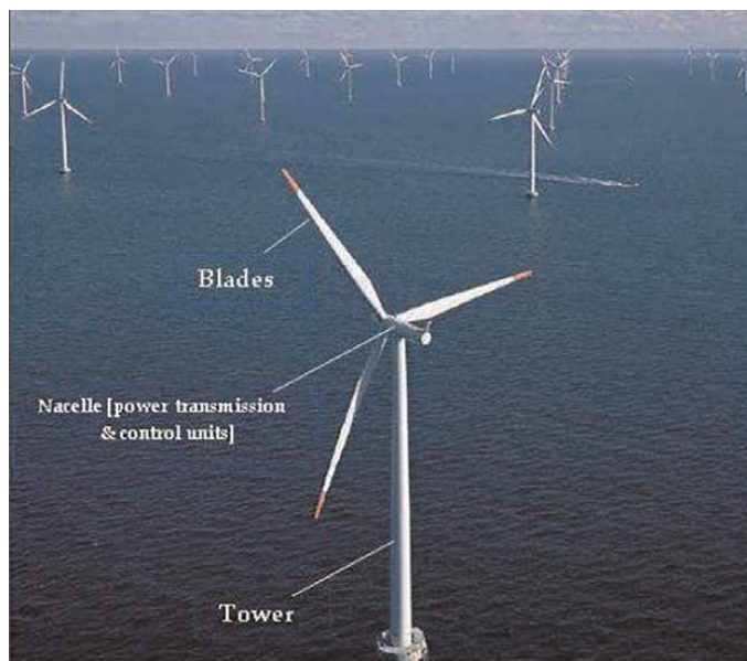
Figure 1. Horizontal-axis wind turbine system components.
