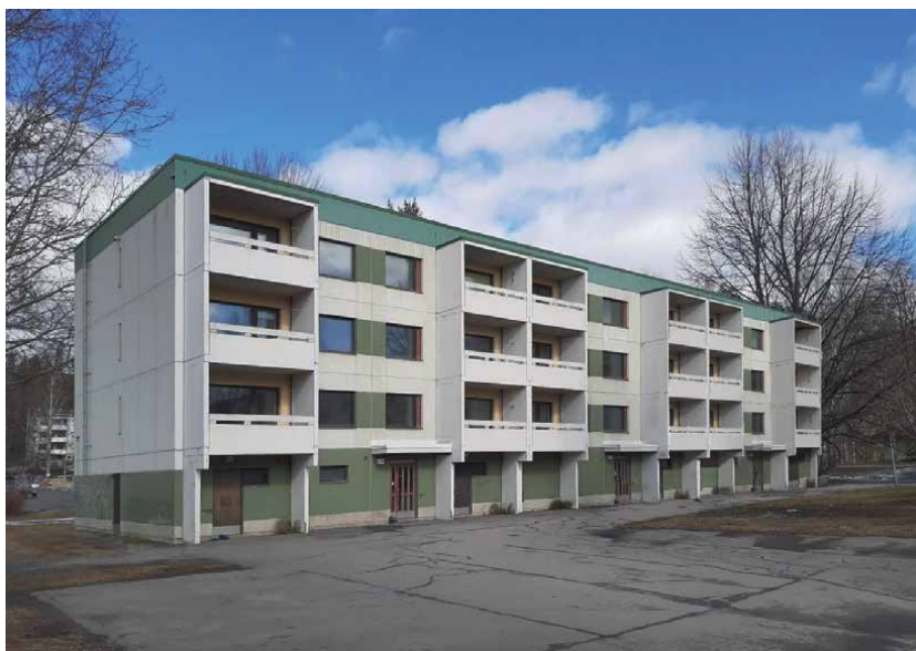
Figure 1. A typical suburban apartment in Finland.
