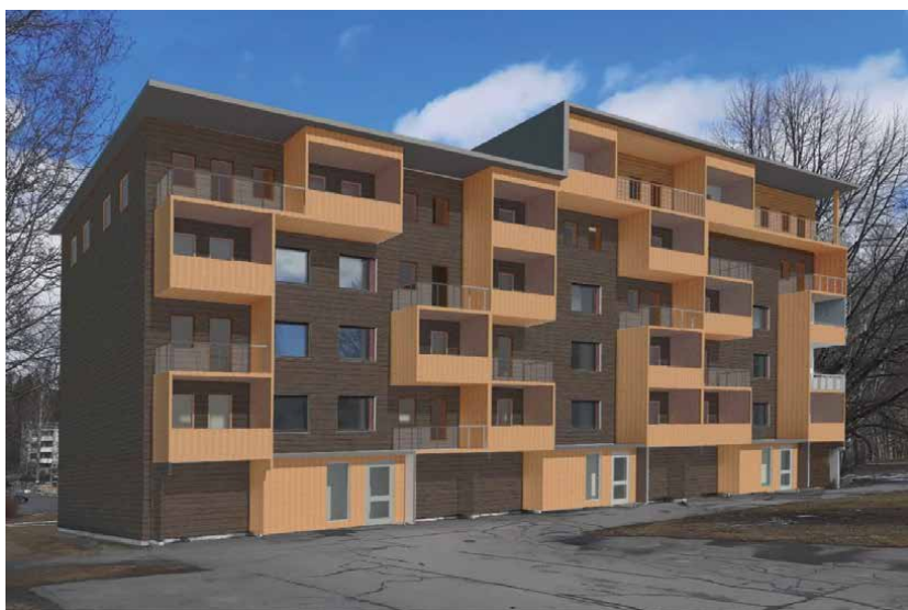
Figure 3. Representative image of wooden facade renovation.
