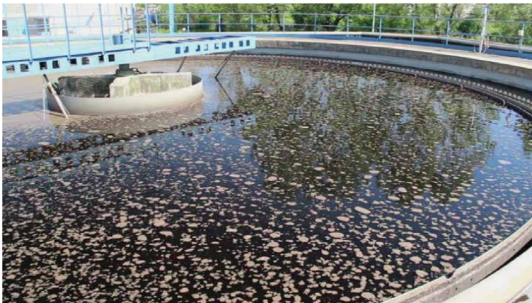
Figure 6. Sewage settling pond.
