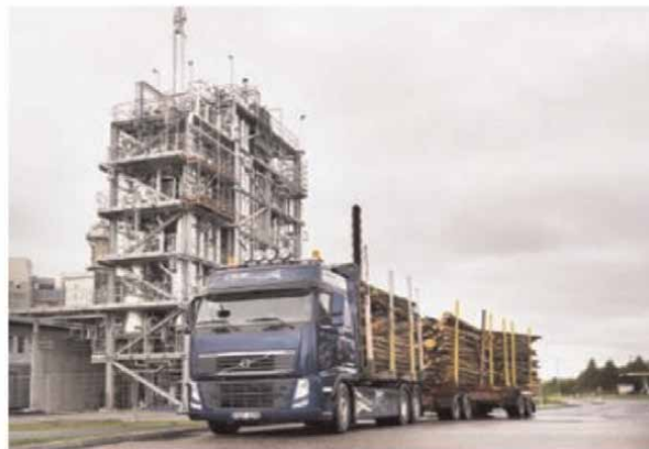
Figure 7. Bio-DME production plant in Sweden [13].
