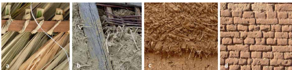
Figure 3. Raw plant fibers in building materials: a-roofing, b-cob and wood, c-cob wall and d-adobe bricks.
