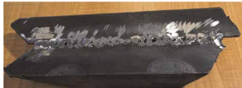
Figure 20. Welds ground-down to remove defects that occurred during the tack welding process joining the two separated pieces.
