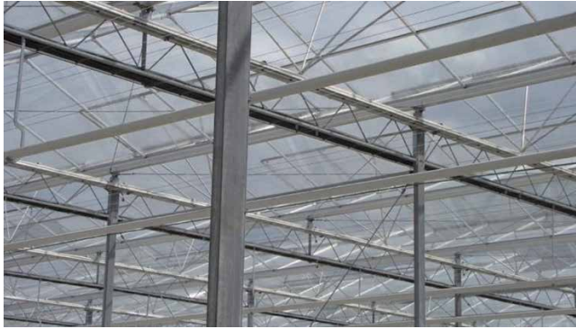
Figure 4. Glass greenhouse-galvanized steel frame (the Netherlands).
