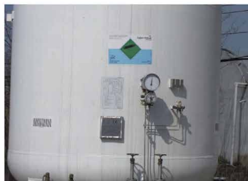
Figure 20. Liquid carbon dioxide tank for supplementing it in the greenhouse (Serbia).
