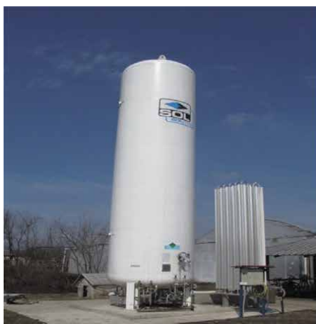
Figure 20. Liquid carbon dioxide tank for supplementing it in the greenhouse (Serbia).
