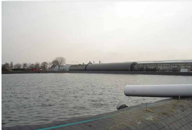
Figure 13. Rainwater pond for the greenhouse irrigation (the Netherlands).
