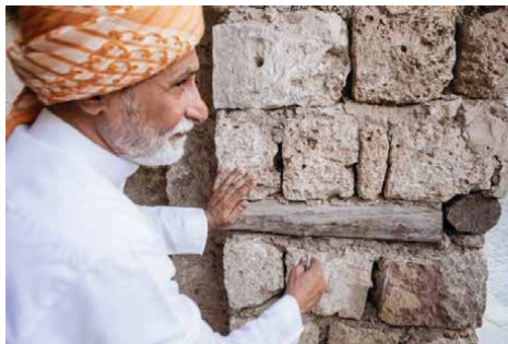
Figure 15. External views of Al-Mangabi blocks and wood beams.
