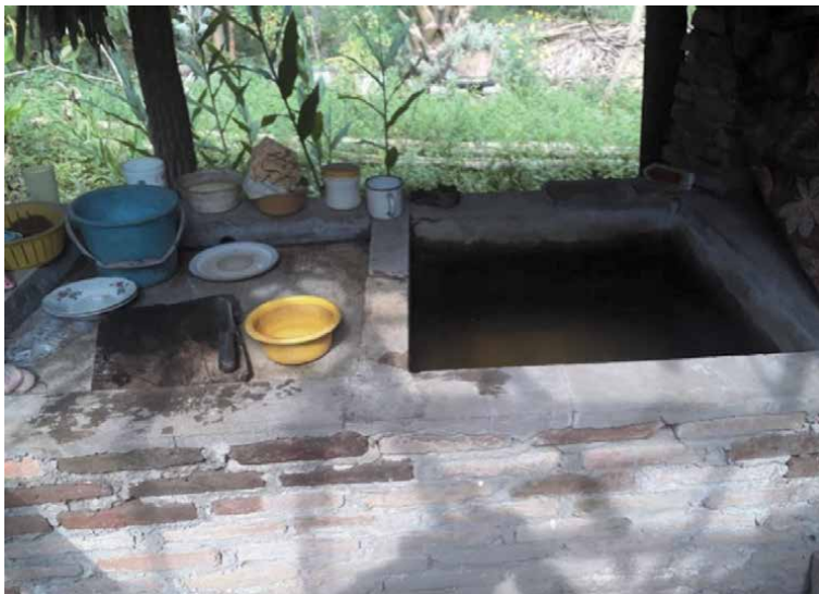
Figure 22. Storage tank features.
