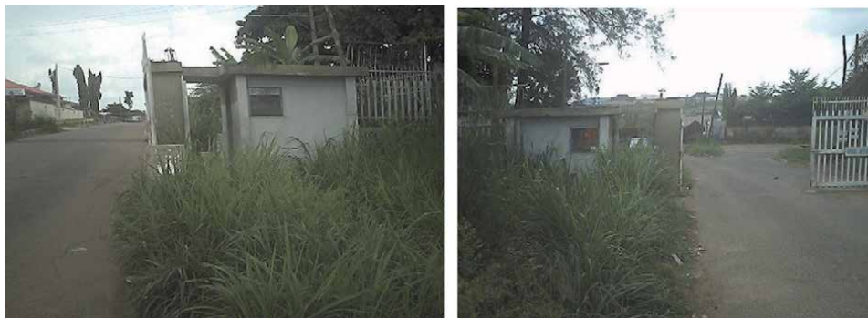
Figure 1. Picture showing the low level of maintenance in the neighbourhood.
