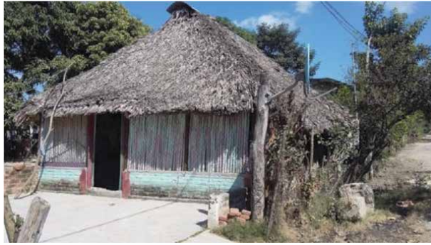
Figure 12. Housing; cane walls and palm roof.
