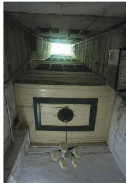
Figure 13. Air shafts in Nasif house (left: Exterior view) and Nawar house (wright: Interior view).
