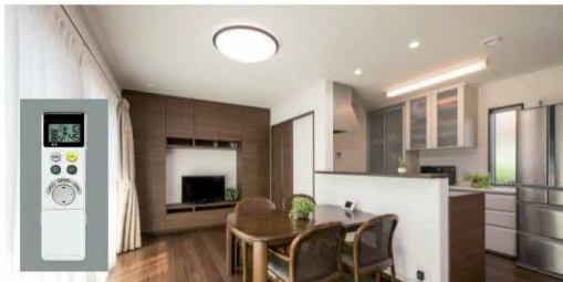
(c) LED lighting fixtures and a lighting control
