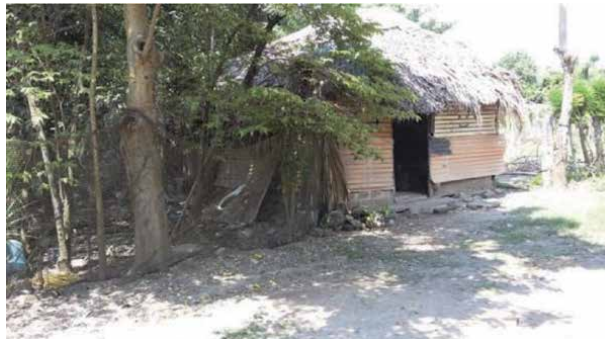
Figure 11. Housing; foil walls and palm roof.
