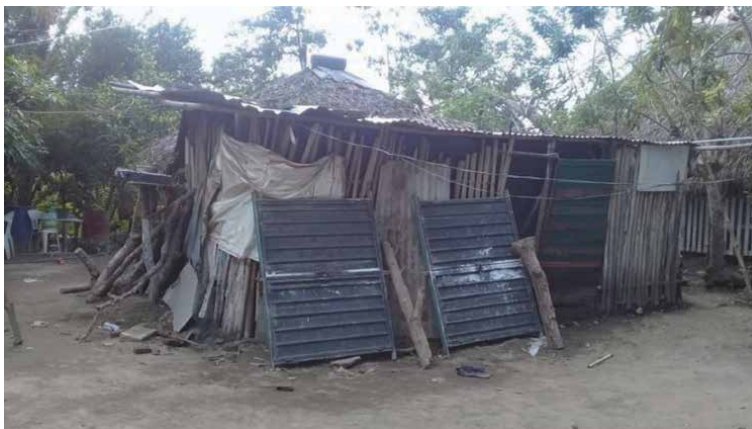
Figure 8. Wooden walls and palm-sheet cover.
