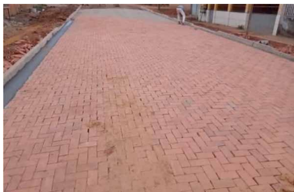
Figure 27. Use of ceramic block as a coating for urban roads with low traffic volume (photo: Jornal AcreAgora ( https://acreaгора.com/2021/07/12/ )).
