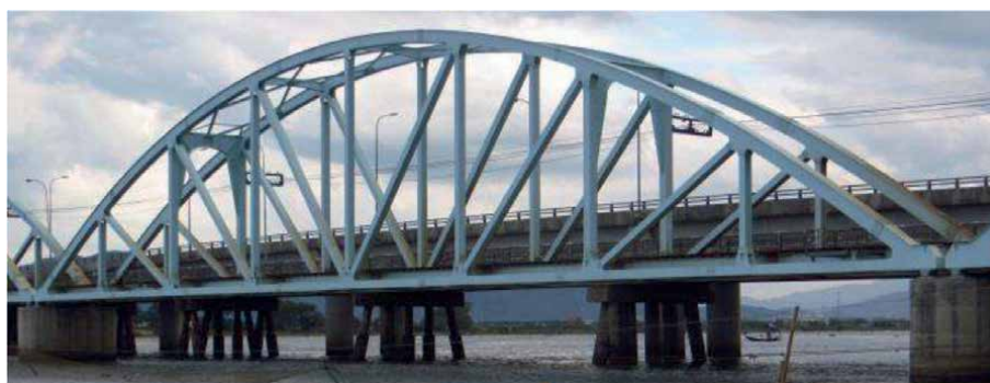
Figure 19. Nam O railway bridge [55].
