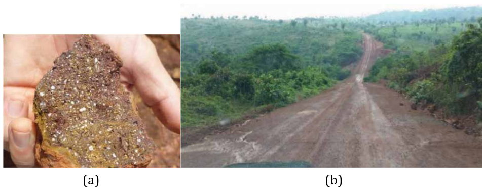
Figure 16. Use of laterites in Amazonian highways. a) Detail of lateritic concretion, with a predominance of iron and aluminum oxides; b) primary coating layer aiming at the durability of the pavement until the execution of the asphalt course (photos: NS Campelo).
