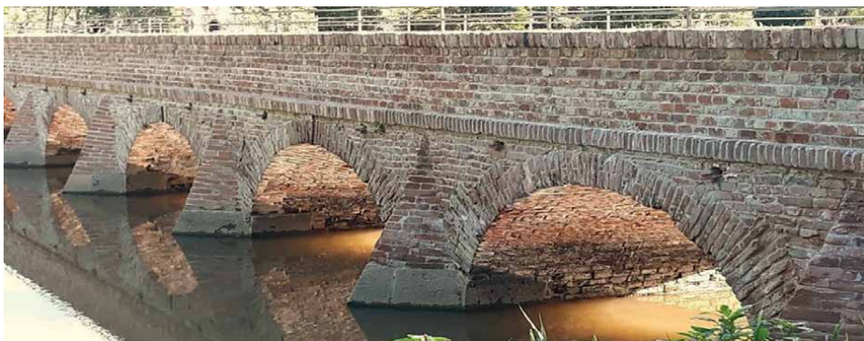
Figure 1. Historic brick bridge.
