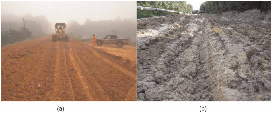
Figure 6. Vicinal roads were built on (a) terra firme (upland area) (lateritic soil), and (b) on várzea (floodplain area) (photos: NS Campelo).
