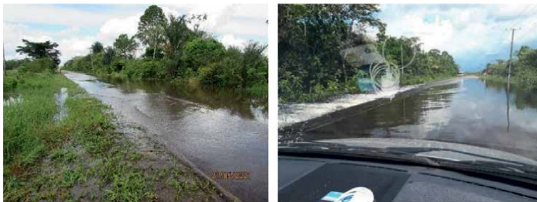
Figure 21. River flooding causing overtopping at some places on federal highway BR-319 (photos: NS Campelo).
