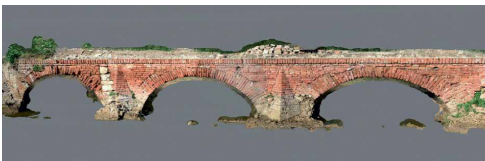
Figure 3. A cut out of the overall 3D model of the bridge created by laser scanning within an archaeological survey in 2019. A later alteration is visible on the first arch from the left, where the extended vault replaced the old wooden drawbridge [2].
