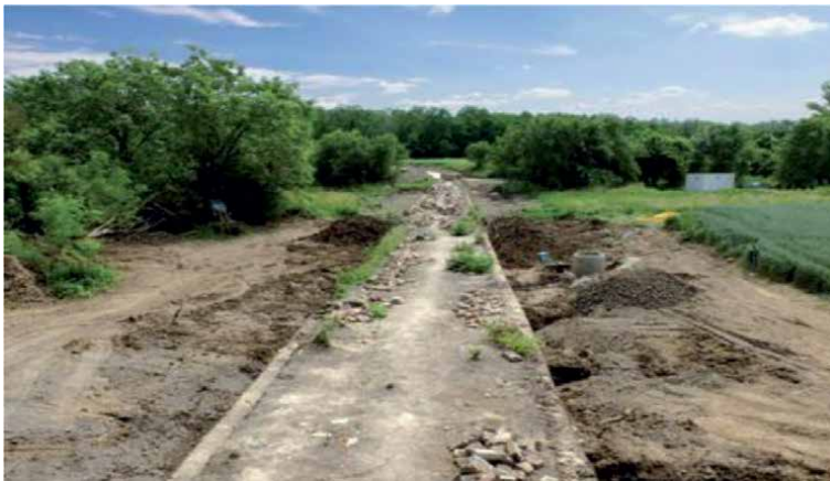
Figure 13. An overall view of the top of the bridge during reconstruction.
