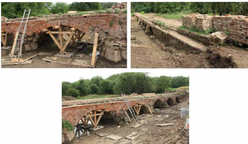
Figure 14. Dismantling and support of arches, summer 2019.
