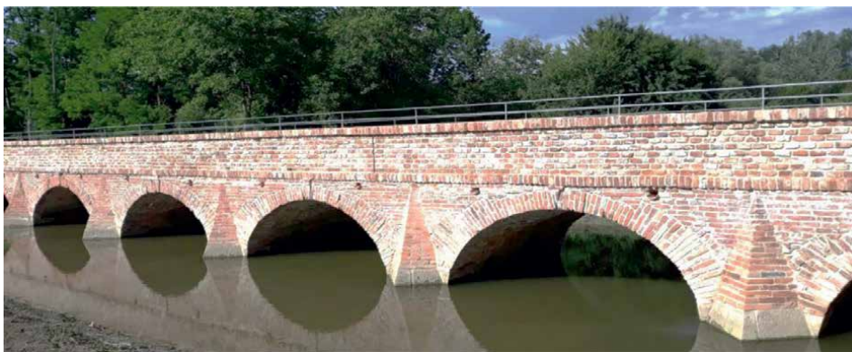
Figure 16. The bridge after completion, 2020.
