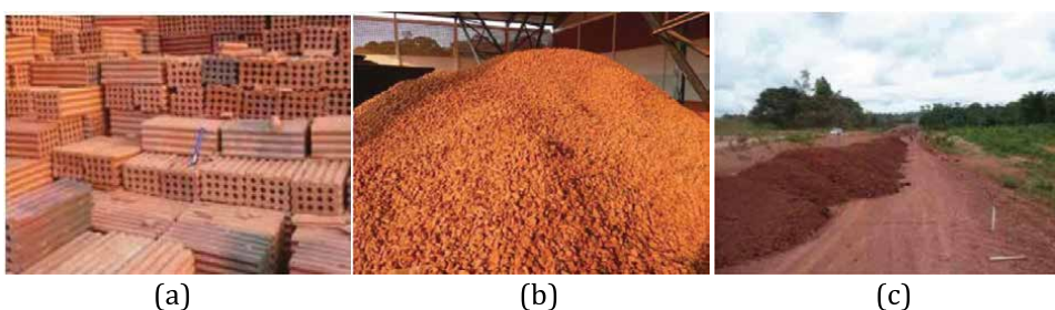
Figure 6. Use of SCACC in highway paving: a) burnt of ceramic bricks following a controlled firing temperature; b) crushing of the ceramic bricks. c) Stacking of the mixture of lateritic soil and SCACC in the field [4].
