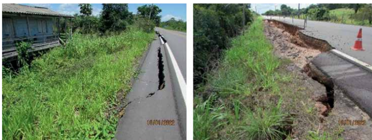
Figure 22. Rupture of road slopes, after the river ebb cycle (photos: NS Campelo).
