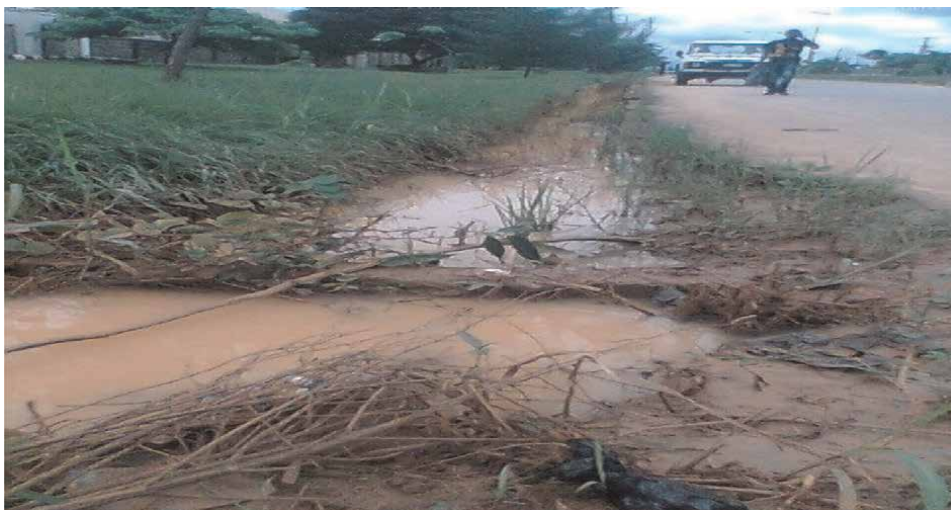
Figure 3. A waterlogged open concrete drain serving as mosquito breeding ground in new Owerri Nigeria.
