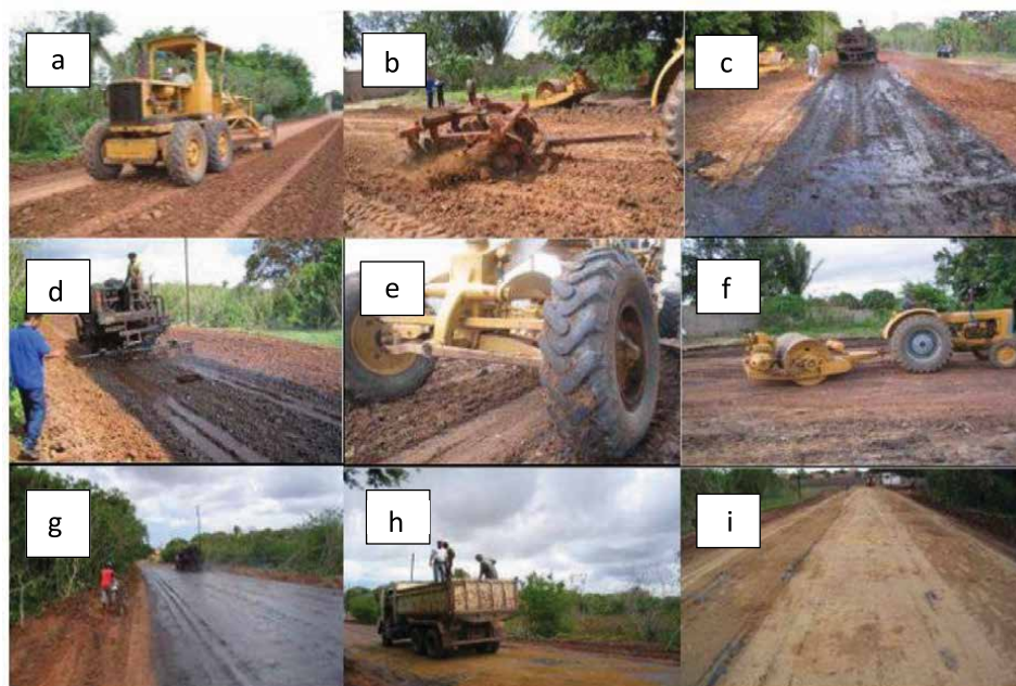
Figure 9. Some records of the execution stages of the experimental section with soil-emulsion [5].
