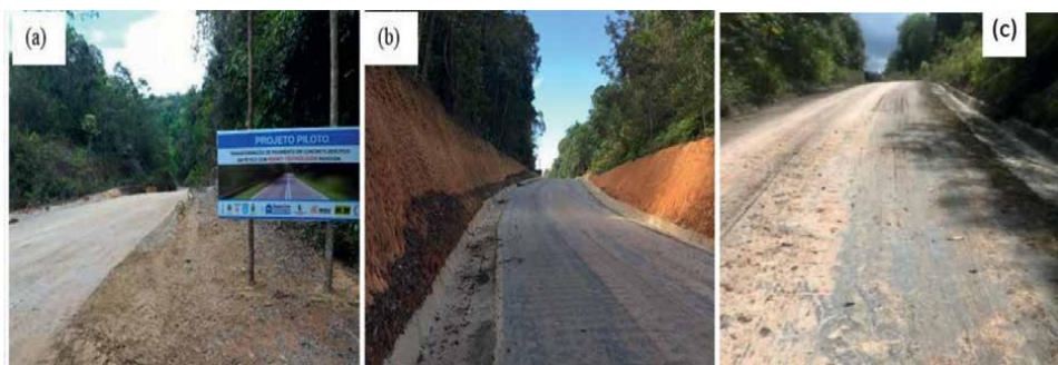
Figure 5. Final aspect of the experimental section. a) One day of stabilization, in Oct. 2016; b) after 490 days, in Feb. 2018; c) after 4 years, Oct. 2020 [1].
