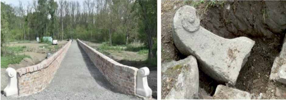
Figure 4. The original quoin stone found before the present restoration of the bridge started. The uncovered fender was used in making replicas during the heritage restoration.
