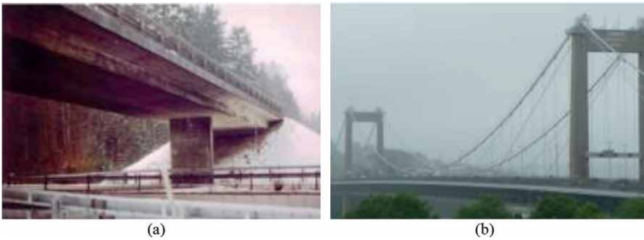
Figure 16. (a) Z24 bridge, and (b) Tamar suspension bridge [52].
