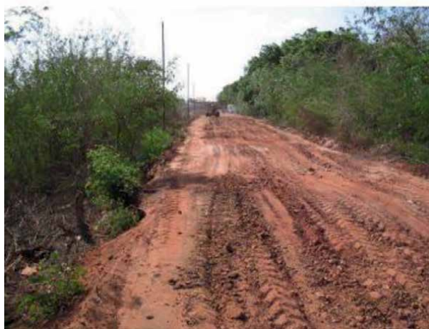
Figure 8. View of the experimental section before stabilization with asphalt emulsion [5].
