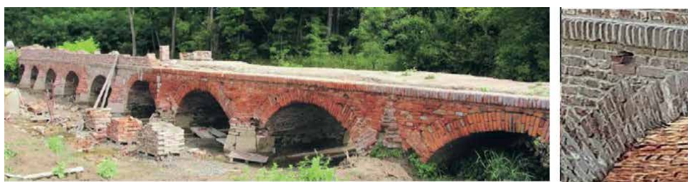
Figure 15. View over the bridge during reconstruction, summer 2019 and detail drainpipes replicas.
