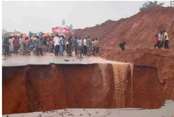
Figure 3. Road cut as a result of soil degradation.
