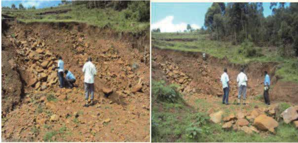
Figure 3. In-situ soil property analysis within the landslide scars. Photo credit, Nseka. November, 2019.
