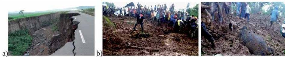
Figure 7. Road collapse at Alem village, Dodota district, along with the Dera-Assela road (a) and mudslide that killed 22 people and domestic animals in Tulu-Gola village, Western Arsi zone (b and c).
