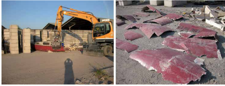
Figure 3. Breaking up of a polyester boat into panels [4].
