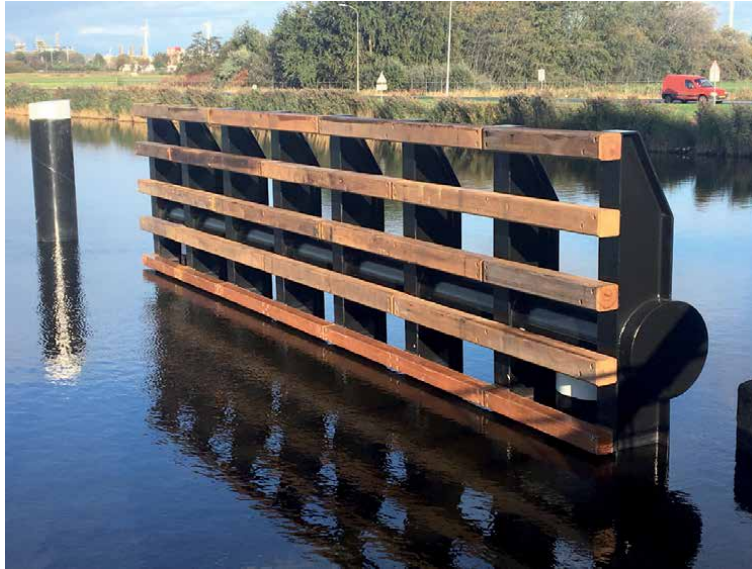
Figure 12. Guiding structure with two lowest rows of beams made from EoL composite [3].
