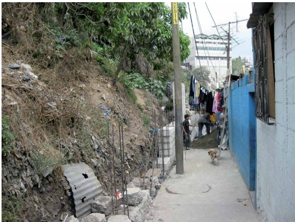
Figure 2. Dwellings have been constructed upon portions of a former landfill using concrete blocks and corrugated metal.
