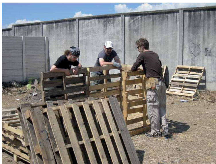
Figure 11. Wooden shipping pallets are readily available and can be simply fastened together to replicate the three-cell compost system.
