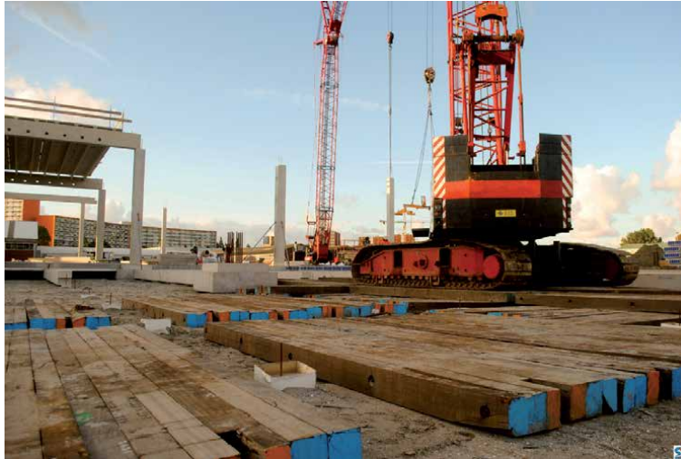
Figure 13. Crane mats in use at a building site [3].
