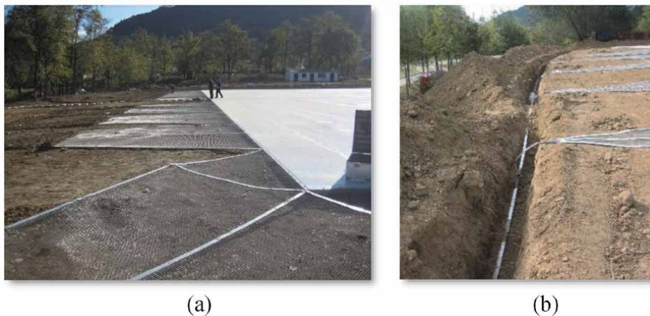
Figure 9. The grounding of the triangular wire mesh. (a) Triangular wire mesh and (b) tip of the triangular wire mesh.
