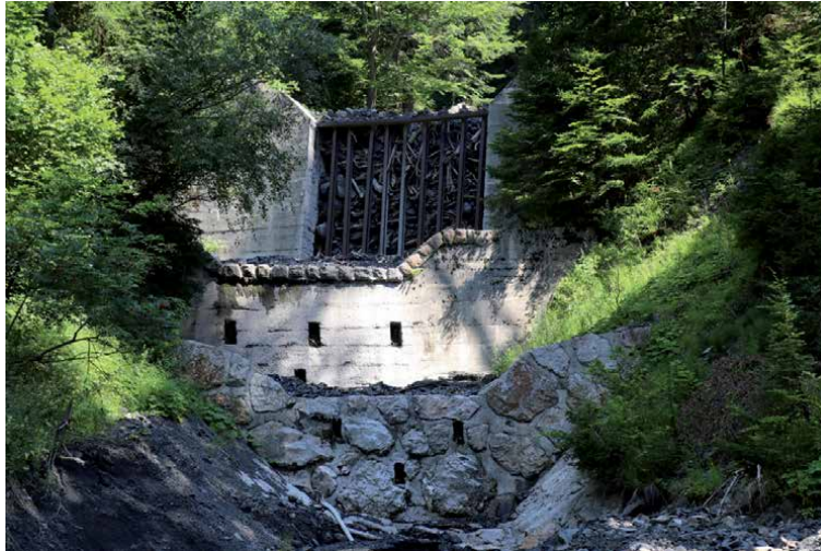
Figure 5. System of torrent barriers on the Suhelj torrent (photo: Jurij Beguš).
