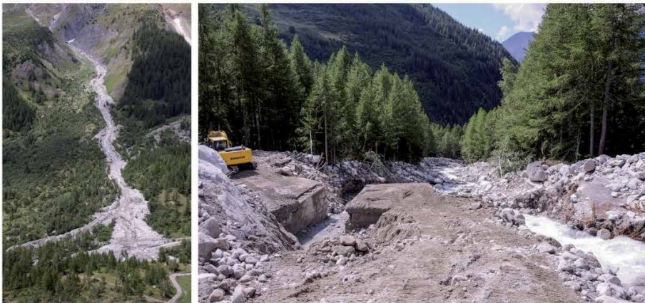
Figure 4. Debris flow deposit in Val Ferret and clearing operations of timber and debris from the stream bed (photo: FMS).
