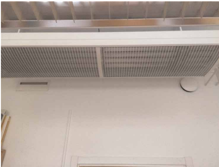
Figure 5. Retrofit of cooling beam (with attached light fixture) leading to a high degree of ventilation short-circuiting. Air supply device to the left and air exhaust to the right.
