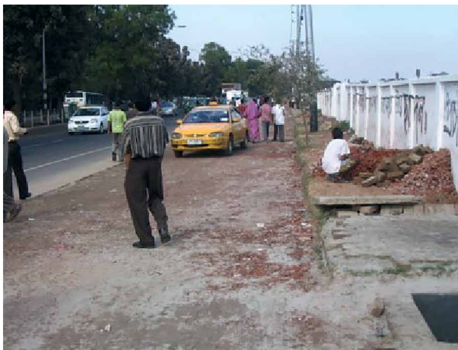
Figure 3. Road widening at the expense of footpaths and shade trees at Sewrapara-Farmgate road under DUTP (source: WBB trust) [20].
