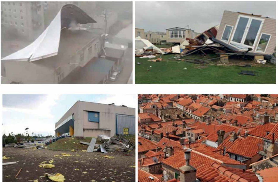
Figure 3. The environment assessment is essential to identify the possible risks and the elements that can fail in case of strong winds, becoming flying debris.
