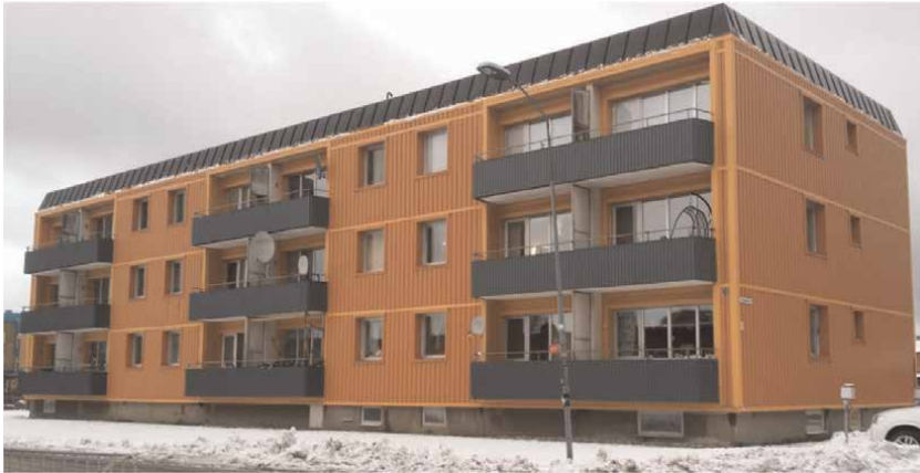
Figure 1. Studied building, Tebogatan 5.
