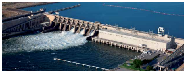
Figure 2. Ice Harbor Lock and Dam, located on the Snake River in southeast Washington State, USA [7].
