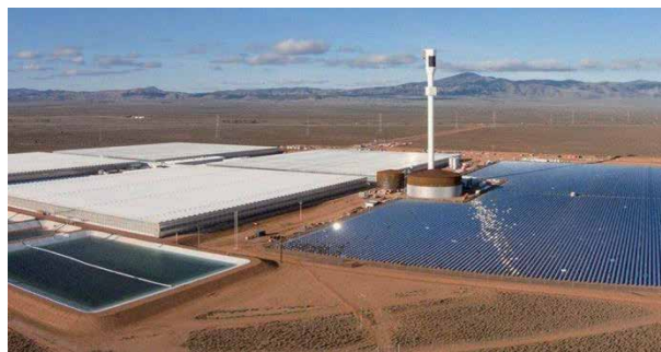
Figure 1. An integrated desalination facility drawing its main electricity from an adjacent concentrating solar power plant [26].
