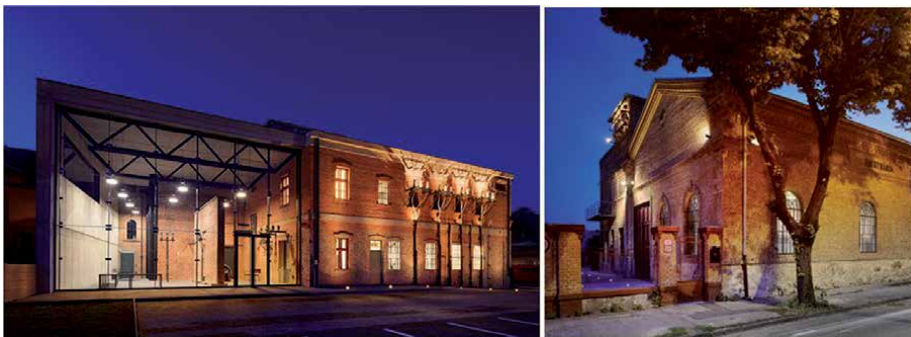
Figure 6. Project of reconstruction of old power plant in Piešťany: M. Ganobjak, V. Hain, M. Paško, Z. Zacharová, 2014 (photo: P. Safko, 2014).
