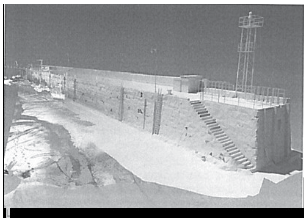
Figure 4. North pier St. Aubins harbour LiDAR screenshot.
