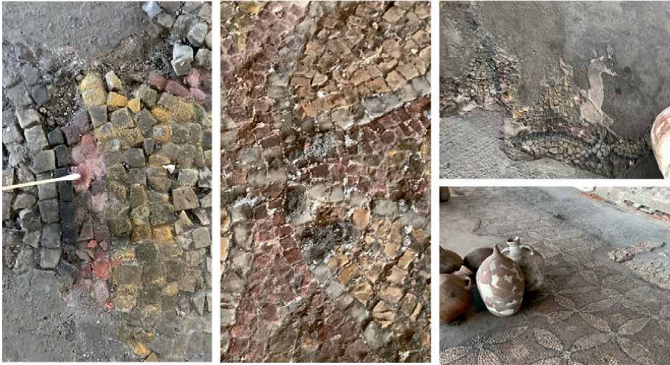
Figure 3. Appearance of the biological attack on tesserae.
