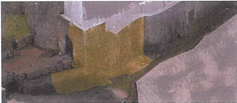
Figure 16. Drone survey of castle. Target area for LiDAR. Screen shots and survey video of castle, Ref. [10], Vid Ref. [2].
