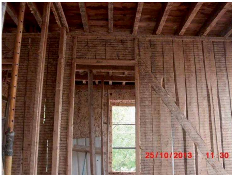
Figure 3. Wood partition wall structure.
