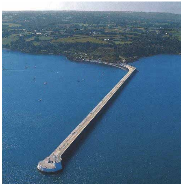
Figure 9. St. Catherine’s breakwater and roundhead 600 m out to sea.
