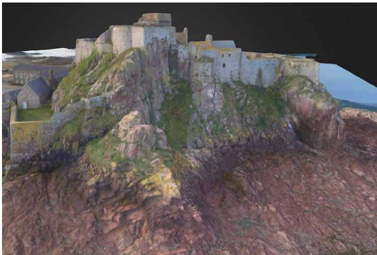
Figure 22. The drone survey model of the higher in accessible west facing castle walls.
