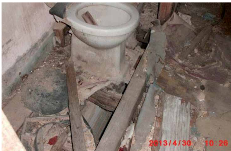
Figure 13. Floor of the Sanit. Installations.
