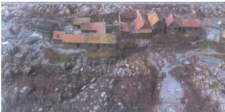
Figure 36. Location of the damaged sea wall to be rebuilt.
