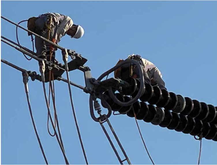
Figure 1. Power line inspection works.
