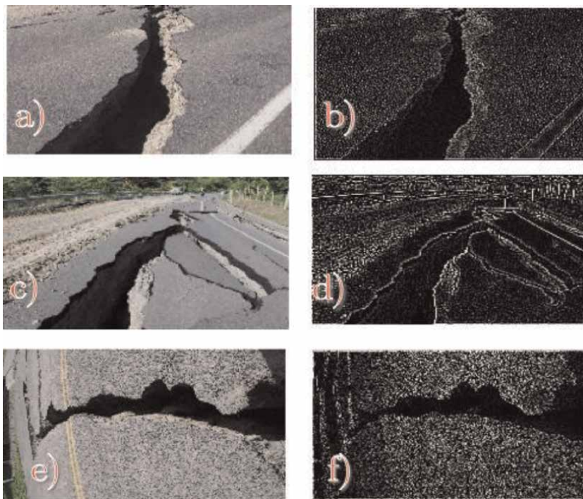
Figure 17. Results obtained by the proposed methodology: a), c), and e) original image, b) and d) processed image (ZZC), finally f) processed image (LC).
