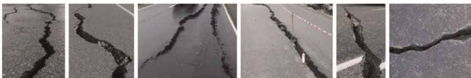
Figure 14. Linear cracks.
