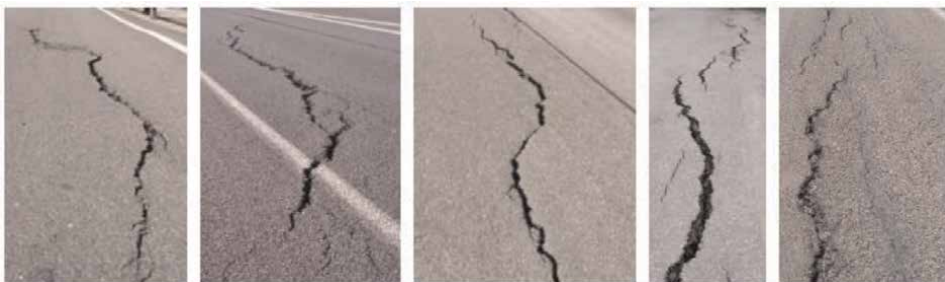
Figure 13. Zig-zag cracks.
