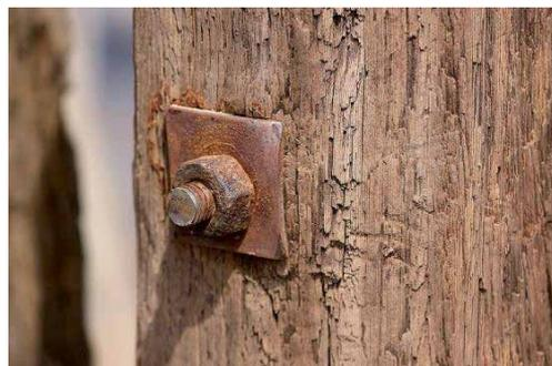
**Figure 2.** Embedded corroded metal fasteners. Source: <https://www.pikist.com/free-photo-socdl/pt>.
