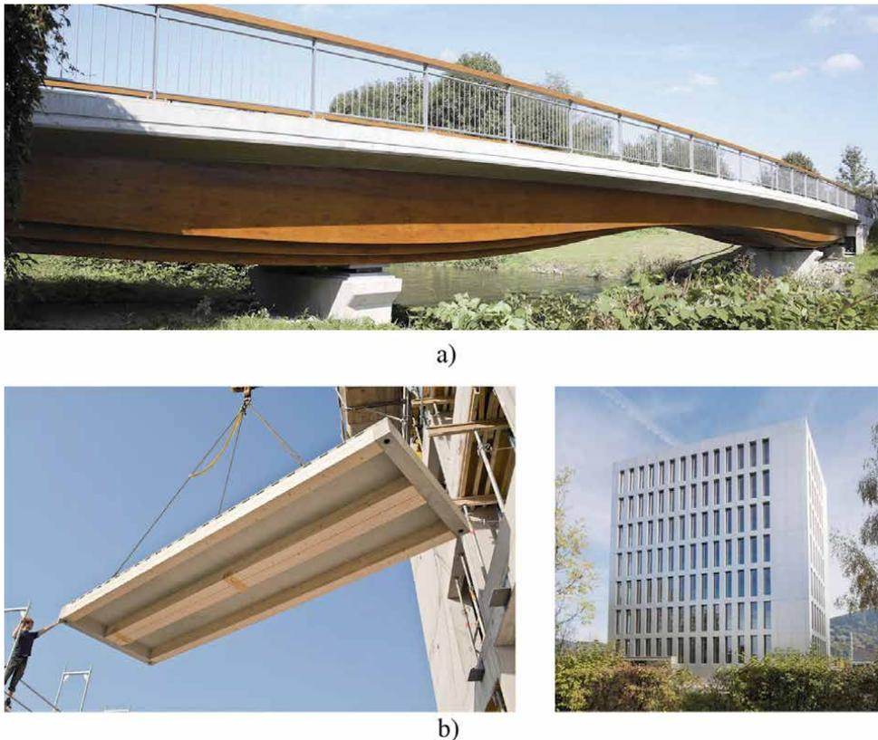
**Figure 1.** Examples of structures with TCC structural elements. (a) Bridge over river Agger, Germany [5]. (b) LifeCycle Tower One, Austria: prefabricated TCC slab during construction (left) and finished building (right) [6].
