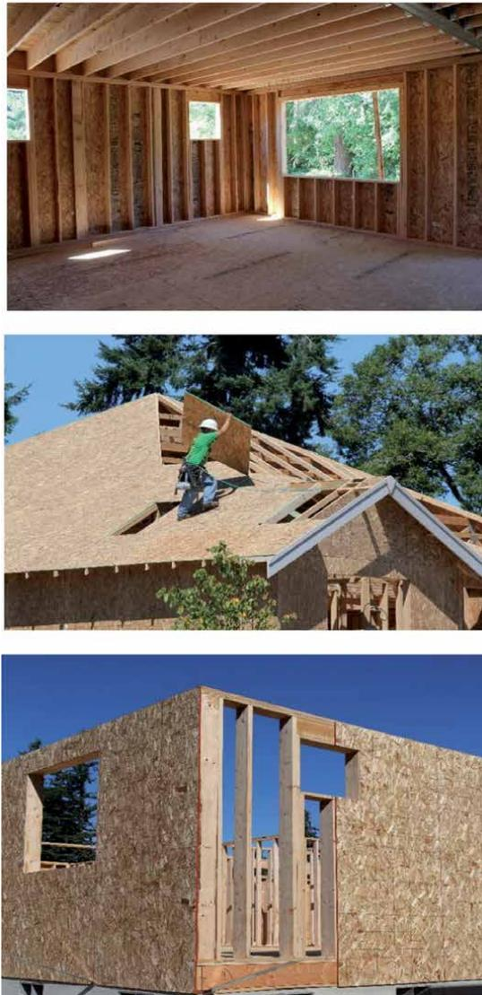
**Figure 5.** OSB sheathing used on floors (top), roofs (center), and walls (bottom) (source: Pictures obtained from APA at <https://www.apawood.org/photography>).
