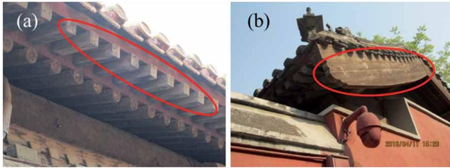
**Figure 7.** The components prone to lightning strike for the ancient building timber. (a) the rafters and (b) the sheathing of Yangxin Hall in the Palace Museum in Beijing (the red ellipse locations highlighted in the figure).
