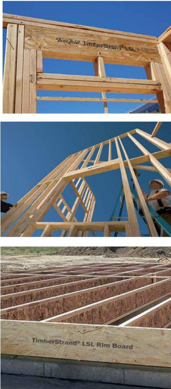
**Figure 12.** Applications of LSL in residential frame construction. Top: LSL header; center: LSL studs; bottom: LSL rim board (source: Pictures obtained from Weyerhaeuser at <https://www.weyerhaeuser.com/woodproducts/>).
