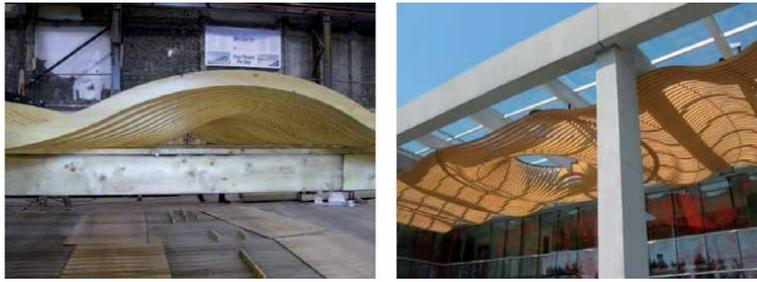
**Figure 10.** Curved LVL structures at Simon Fraser University (Canada) - Ripple Cone Canopy (source: photos obtained from StructureCraft [44]).
