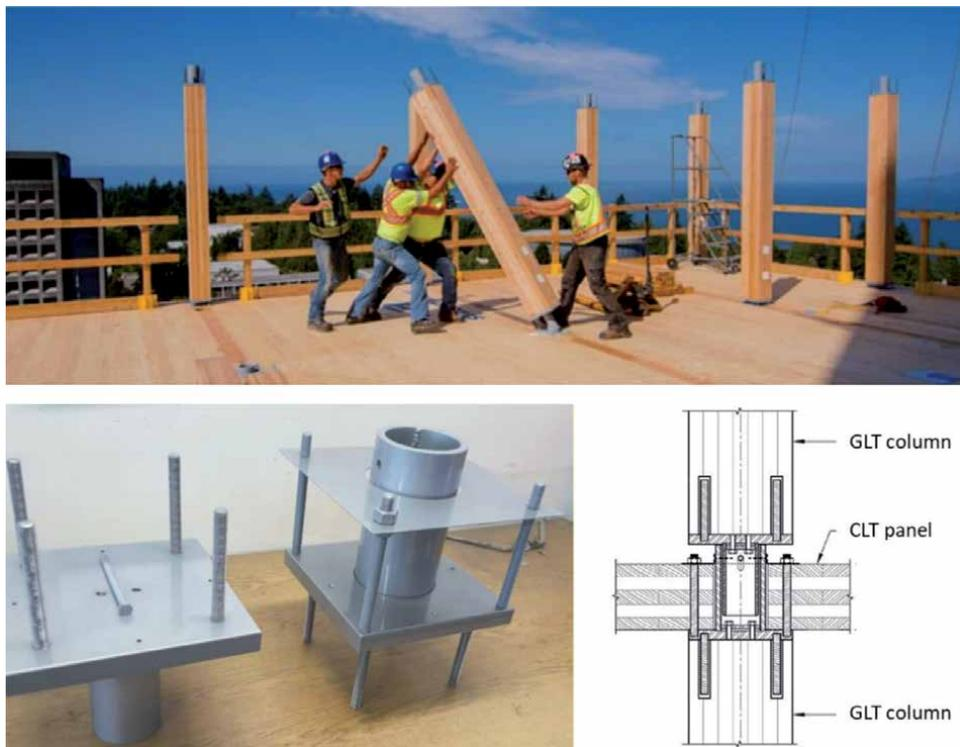
**Figure 19.** Column-to-column connection used in the Brock Commons Tallwood House in the University of British Columbia, Vancouver, Canada (upper: on-site installation of columns connected to CLT panels (source: [www.fastepp.com](http://www.fastepp.com)); lower: HSS steel connectors [26]).
