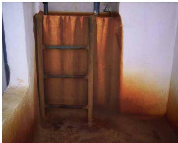
**Figure 4.** *A tank containing iron-rich water. Iron ions can be present in the aqueous phase either from the corrosion of metallic parts or they may be present in groundwater at concentration levels depending on the mineral composition of the aquifer.*
