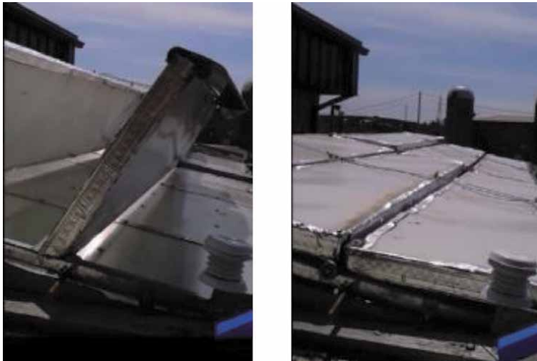
Figure 6. Opening (right) and closing (left) of the CING rooftop panels.
