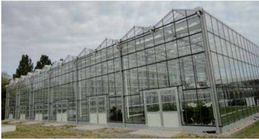
Figure 1. Multi-span Venlo glass greenhouse in Hannover, Germany.
