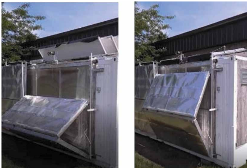
Figure 5. Opening (left) and closing (right) of the CING insulating panels.
