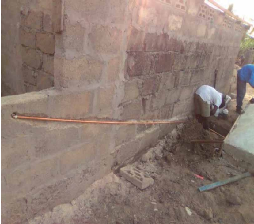
Figure 8. Installation of galvanised copper pipes for tapping biogas into kitchen.
