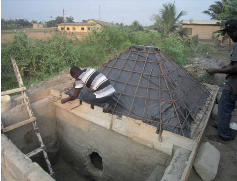
Figure 3. Construction of a pyramidal-shape biogas digester insulated with black polythene bag.
