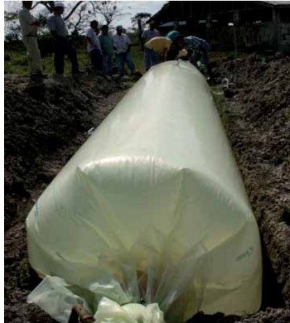
Figure 4. Example of low-cost PE- digester installation in South America. Image courtesy: Shikun Cheng.
