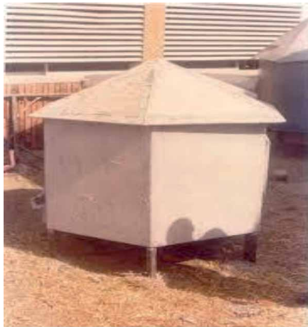
Figure 14. A 1.4 m 3 capacity wooden grain silo. Source [43].
