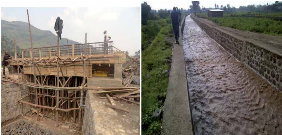
Figure 12. Construction of bridge and river drainage canal. Source: GWLM project.
